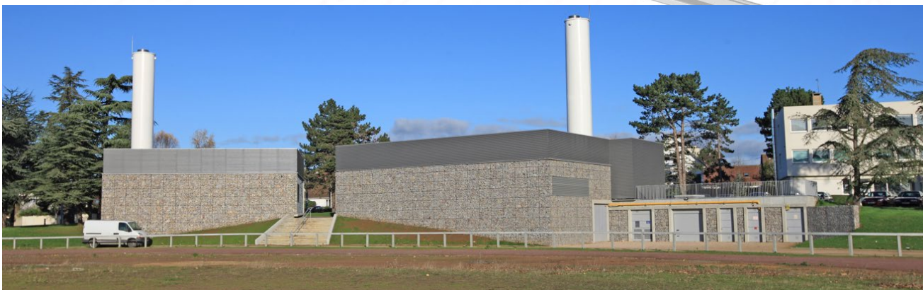
Chaufferie Biomasse Campus 1
